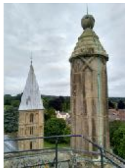
Similar pinnacle on the central tower today
